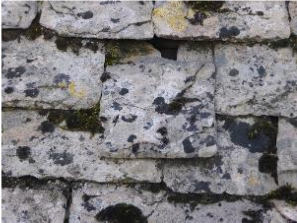
Delaminating and slipping stone slates - North side
