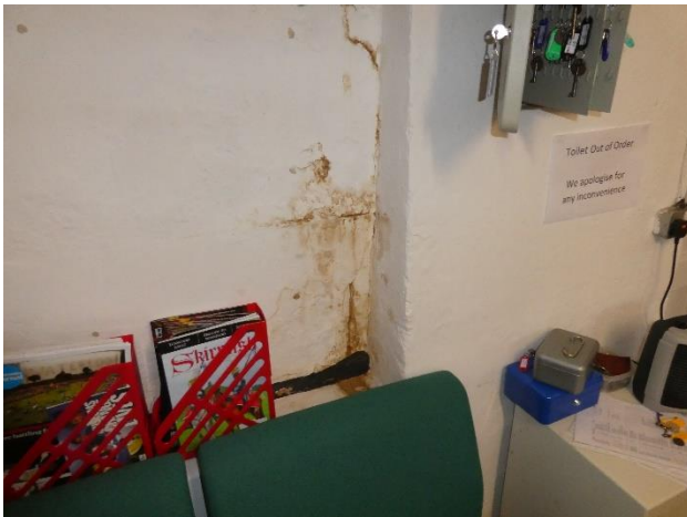
Water damage from leak to Office north wall.
