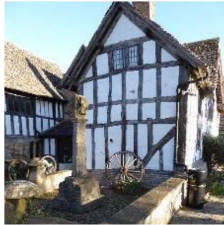
West wall to Office and demolished stable
