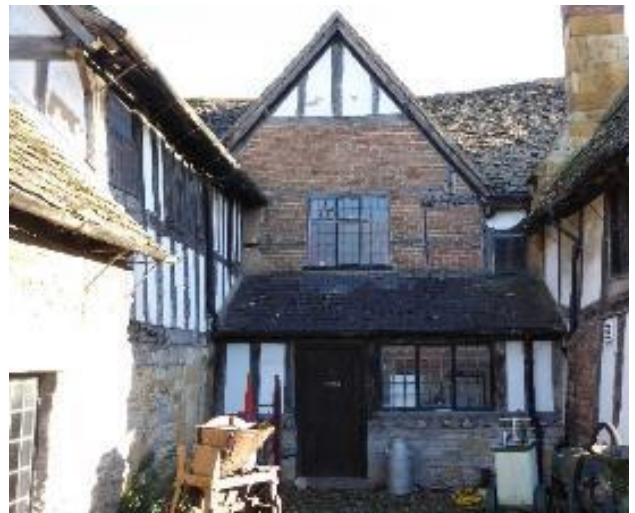
Decaying and possibly blocked downpipe and shaling roof to north side.
