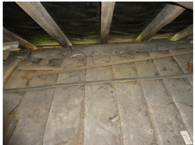
Main attic- Fallen render to west gable forming holes.
