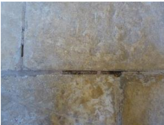
Water damage from leak to Office north wall.
