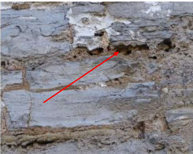
Masonry bee damage - North side.
