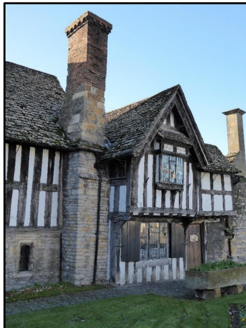
View from the north- east
