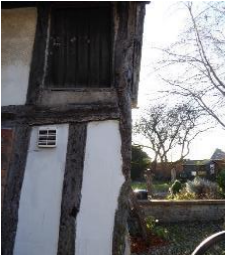
Decaying and racking timber framing to Office wing
