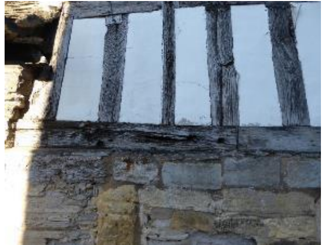
Decaying framing and cracked panels to south main wing
