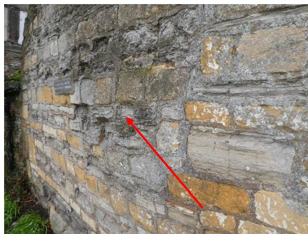
Chimney to north west corner- Stone decay and structural cracking at low level
