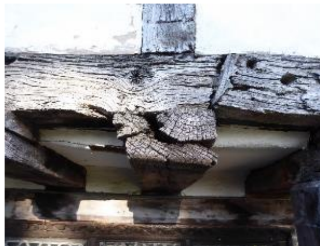
Decaying framing and cracked panels to south main wing
