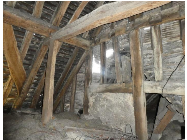
Main attic- Fallen render to west gable forming holes.
