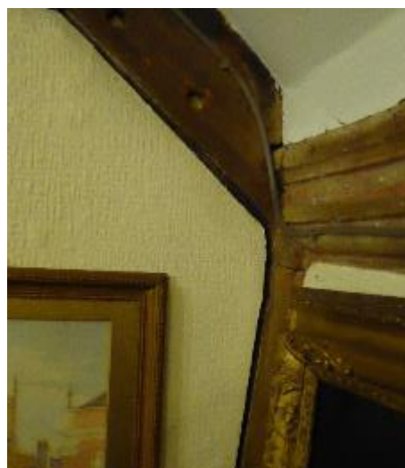
Civic Room Chimney- Tell-tale to cracking to stonework arrowed.
