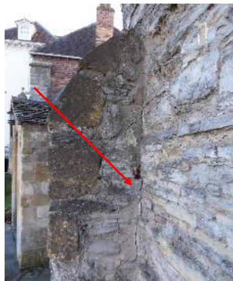
Stone decay to buttress - North side
