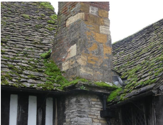
Delaminating and slipping stone slates - North side
