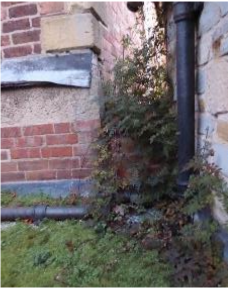
Flat roof over Information Centre
