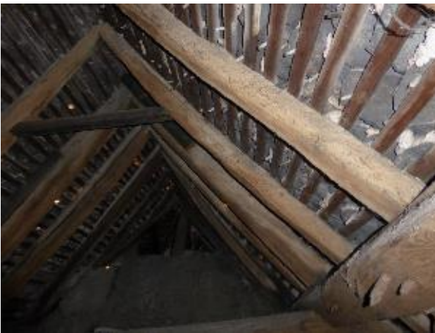
General view of main attic. Note holes in slates.
