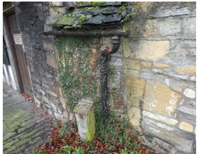
Decaying and possibly blocked downpipe and shaling roof to north side.
