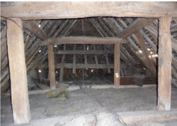
General view of main attic. Note holes in slates.
