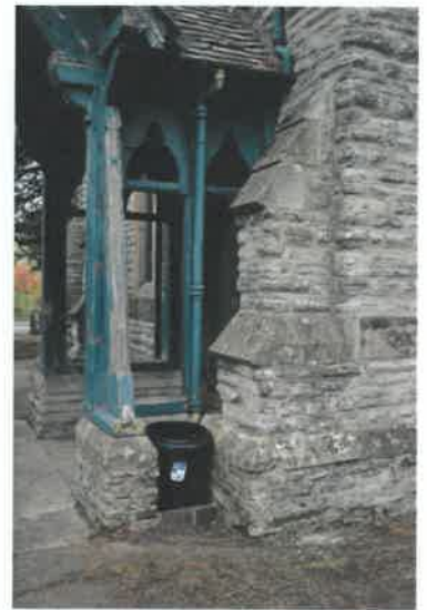
Arcade from south at east chapel
