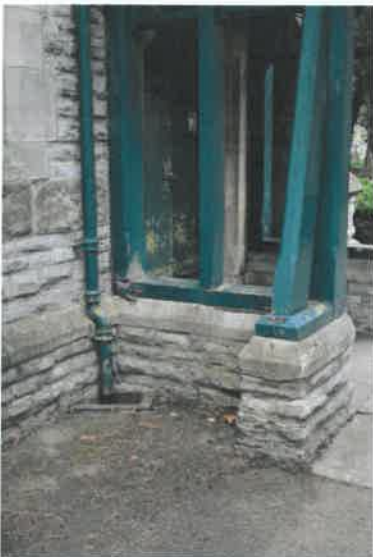
Arcade from north at east chapel
