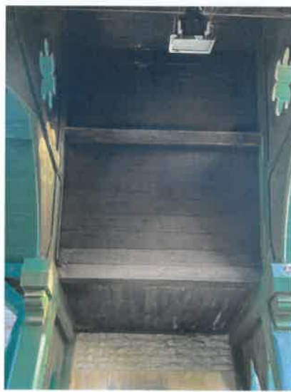
Arcade roof from underside
