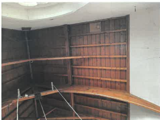
East roof at south bay
