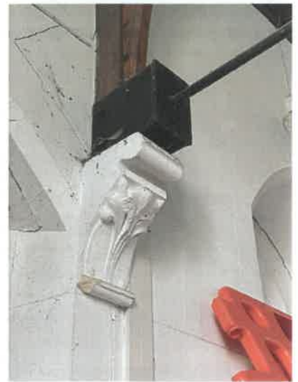
East chapel west wall truss support
