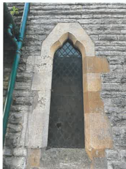
West Chapel east wall window W7
