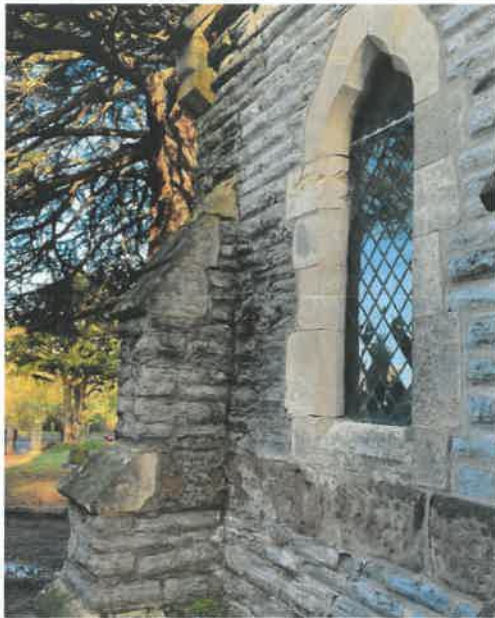
East Chapel west wall
