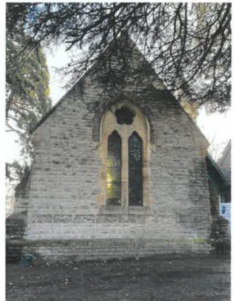
East Chapel north wall
