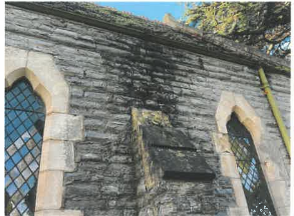
East Chapel west wall
